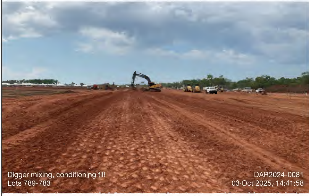
Photo 110 - DAR2024-0081_2025-10-03_Digger mixing, conditioning fill_14-41-58
