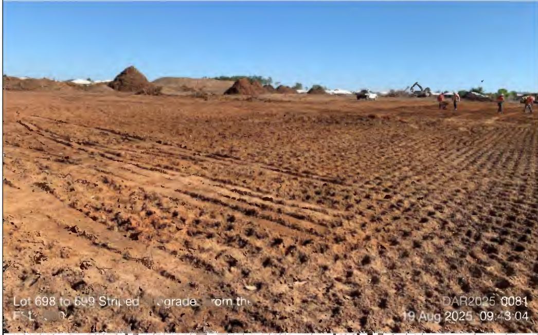
2025-0081_2025-08-19_Lot 698 to 699 Striped subgrade. From the FSL -500
