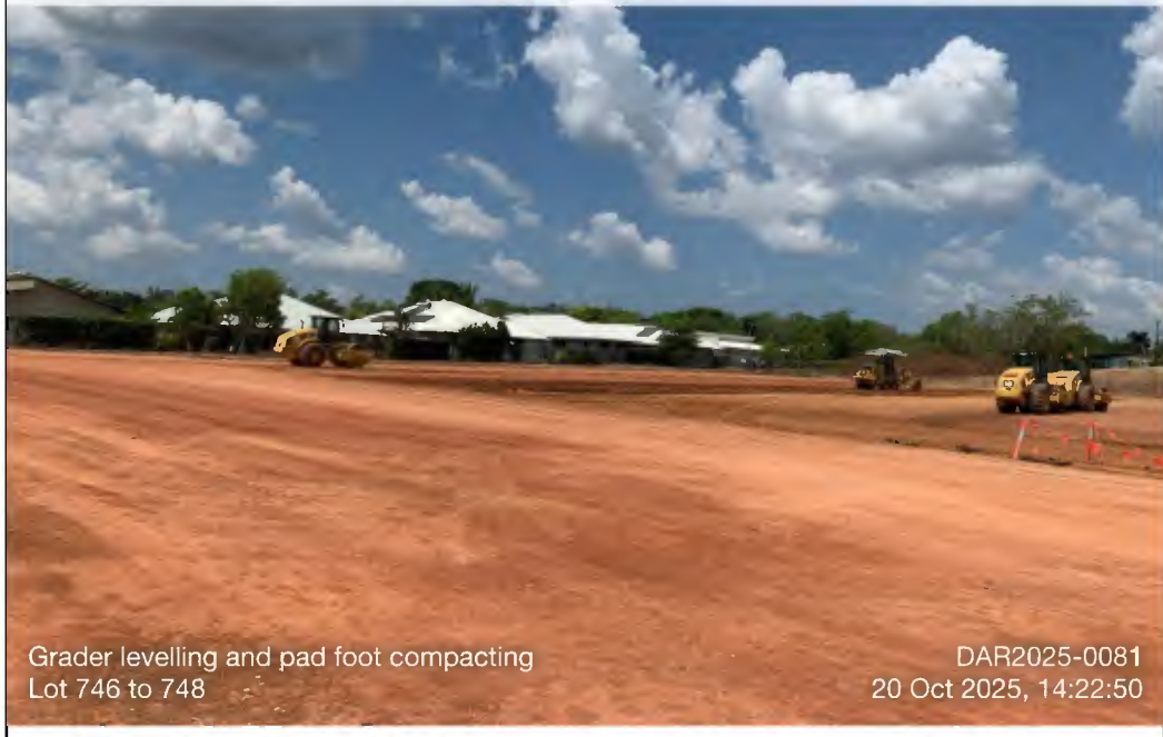
Photo 128 - DAR2025-0081_2025-10-20_Grader levelling and pad foot compacting Lot 746 to 748_14-22-50
