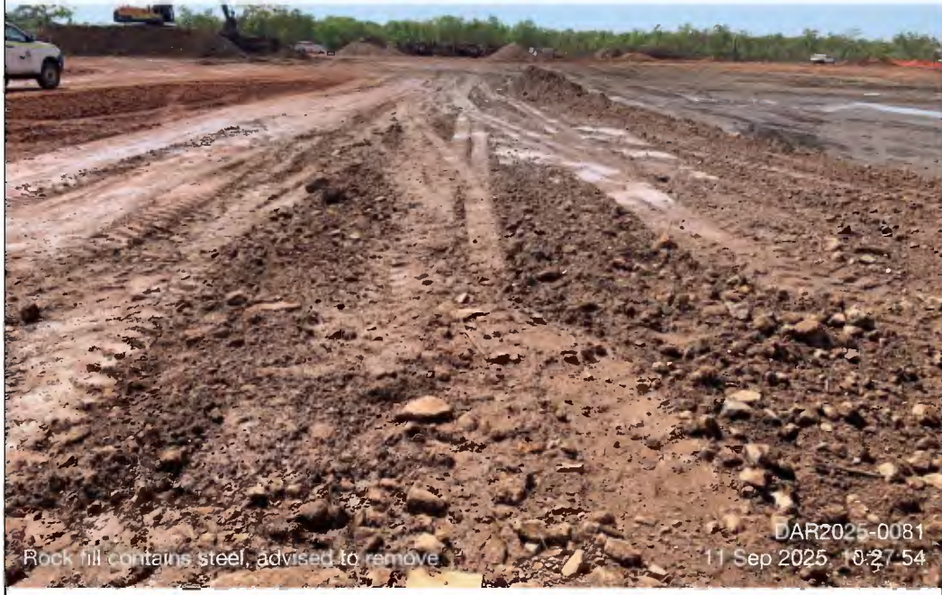
Photo 60 - DAR2025-0081_2025-09-11_Rock fill contains steel, advised to remove._10-27-54
