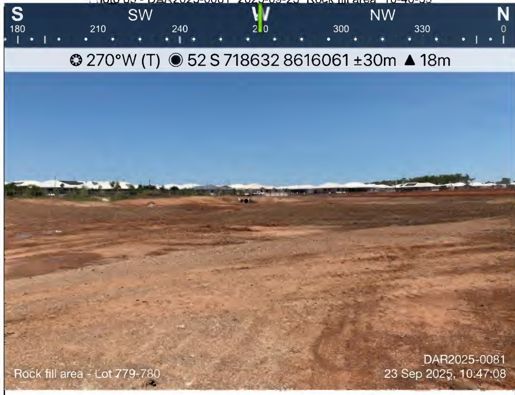
Photo 86 - DAR2025-0081_2025-09-23_Rock fill area - Lot 779-780_10-47-08
