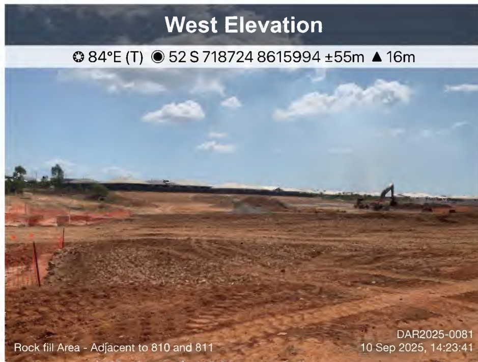
Figure 11: Rock fill placement within deep fill Area (Lot810 and 811)
