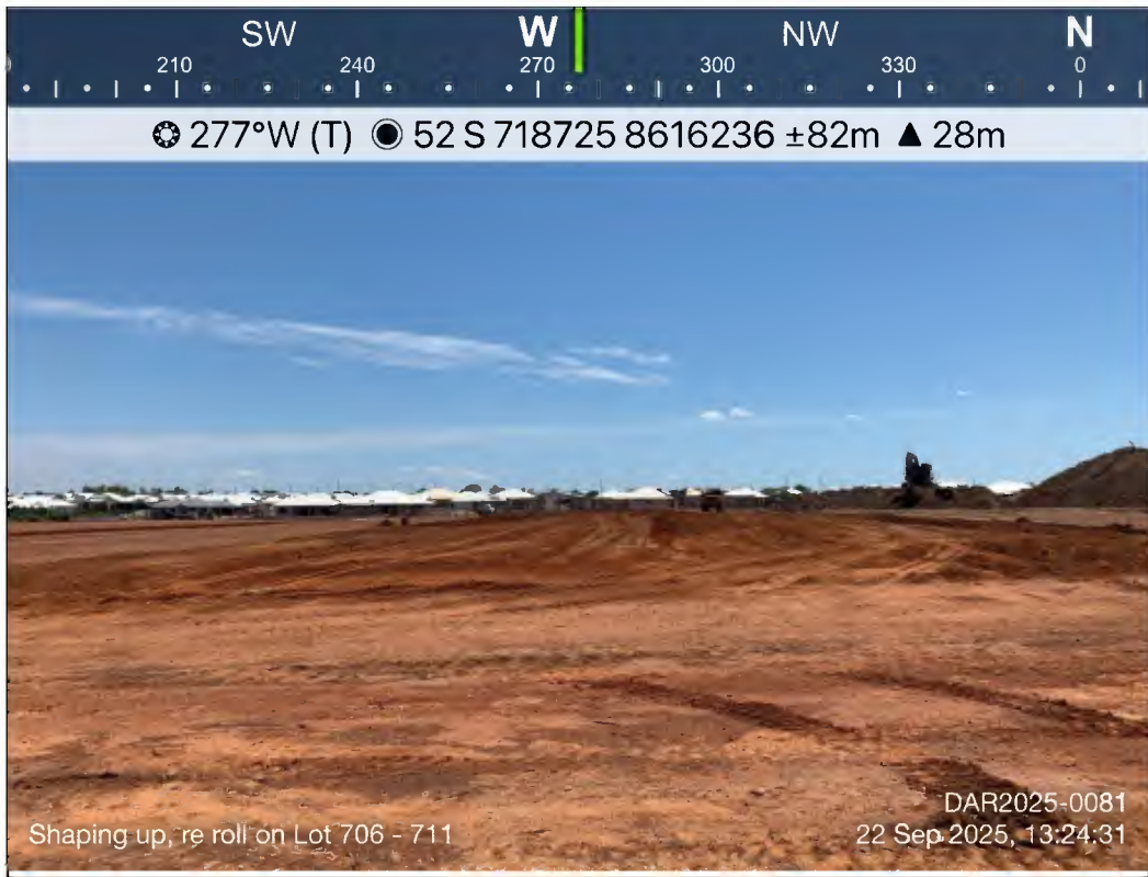
- DAR2025-0081_2025-09-22_Shaping up, re roll on Lot 706 - 711
