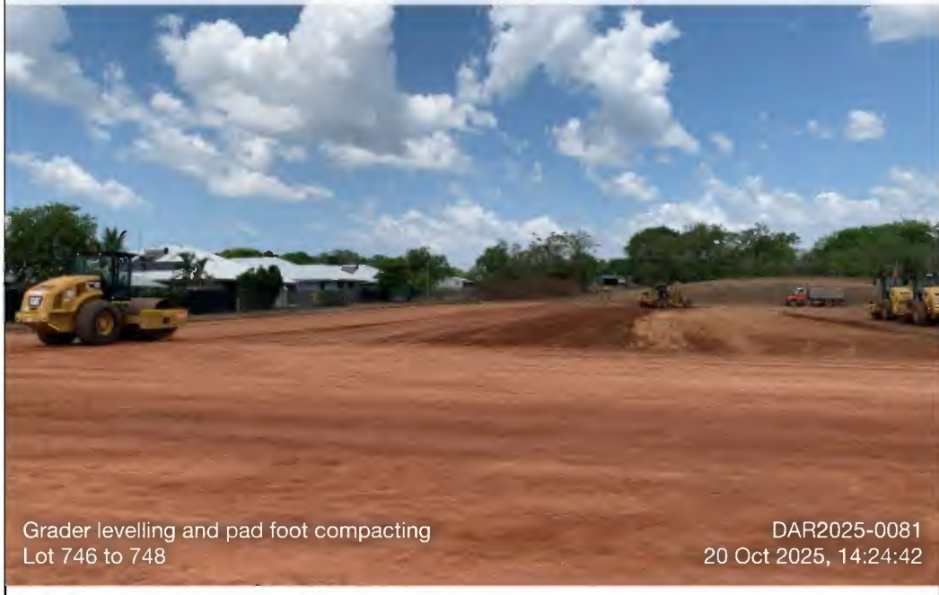
Photo 130 - DAR2025-0081_2025-10-20_Grader levelling and pad foot compacting Lot 746 to 748_14-24-42
