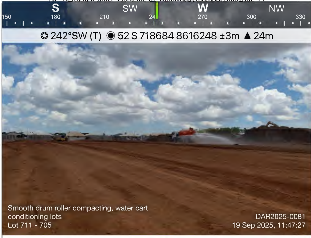
Photo 74 - DAR2025-0081_2025-09-19_Smooth drum roller compacting, water cart conditioning lots_11-47-27
