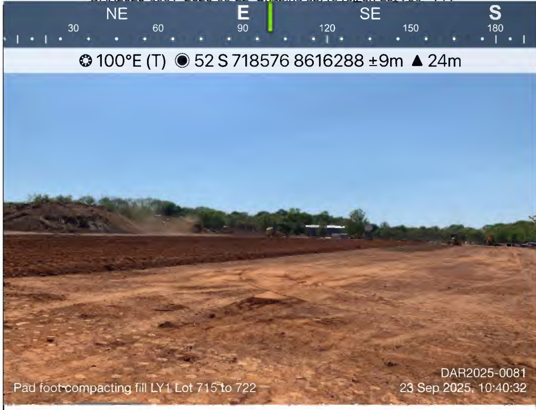
Photo 84 - DAR2025-0081_2025-09-23_Pad foot compacting fill LY1 Lot 715 to 722_10-40-32
