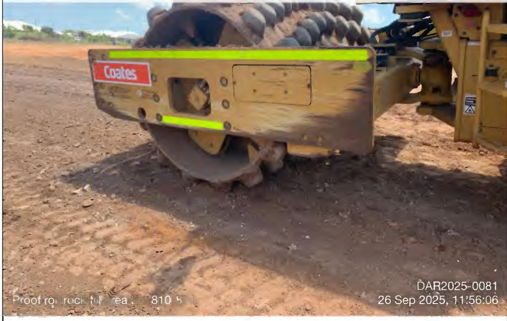
Photo 92 - DAR2025-0081_2025-09-26_Proof roll rock fill area Lot 810-811_11-56-06
