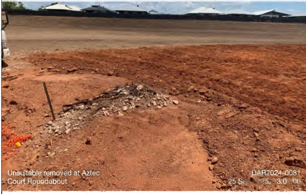
Photo 90 - DAR2024-0081_2025-09-25_Unsuitable removed at Aztec Court Roundabout_13-01-00
