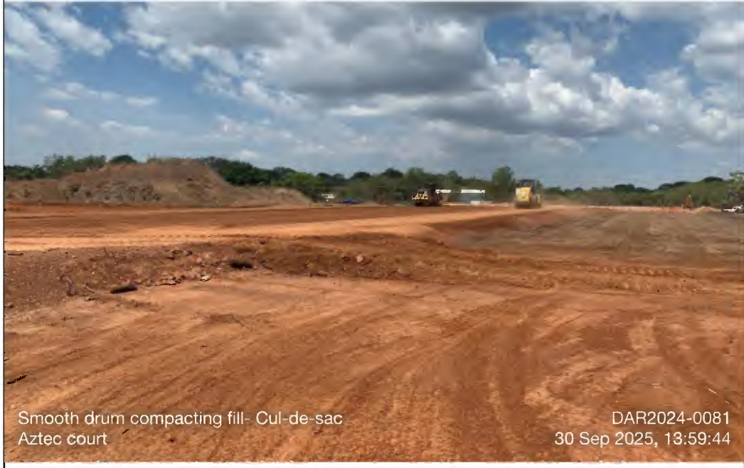
Photo 102 - DAR2024-0081_2025-09-30_Smooth drum compacting fill- Cul-de-sac Aztec court_13-59-44
