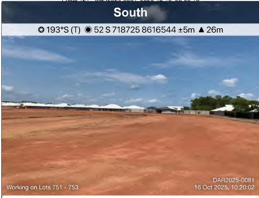
Photo 122 - DAR2025-0081_2025-10-16_Working on Lots 751 - 753_10-20-02
