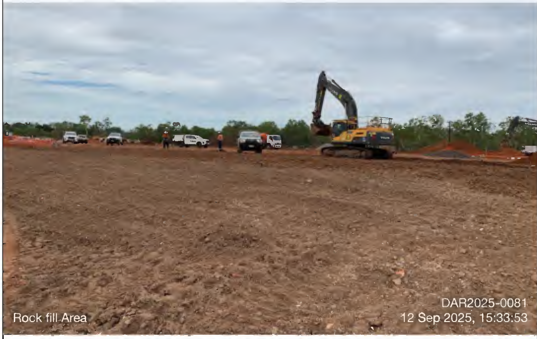
Photo 66 - DAR2025-0081_2025-09-12_Rock fill Area_15-33-53
