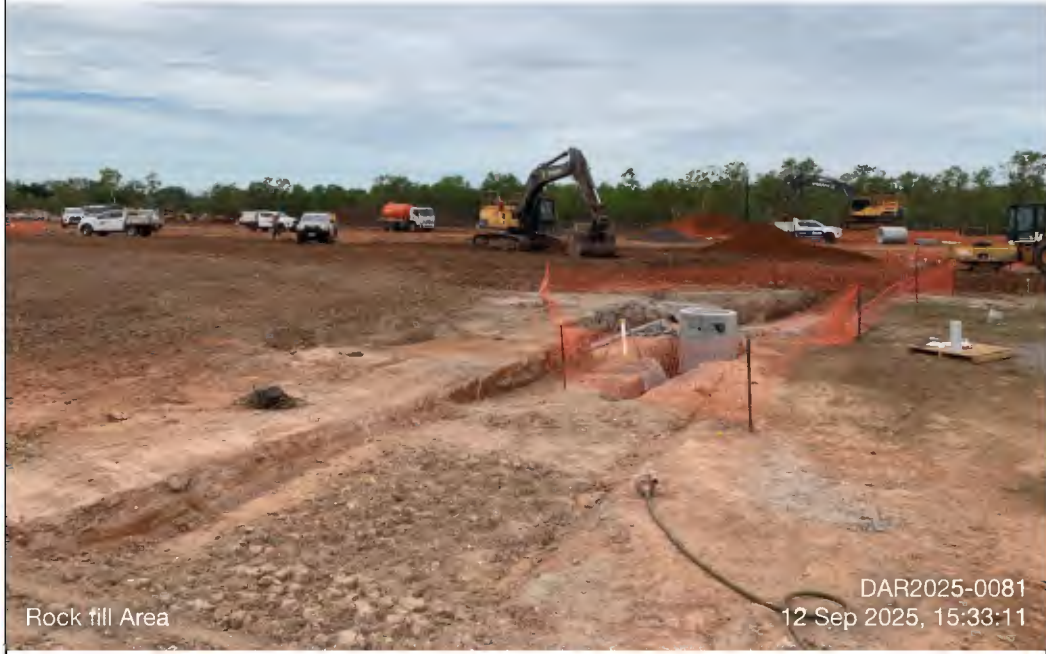
Photo 65 - DAR2025-0081_2025-09-12_Rock fill Area_15-33-11
