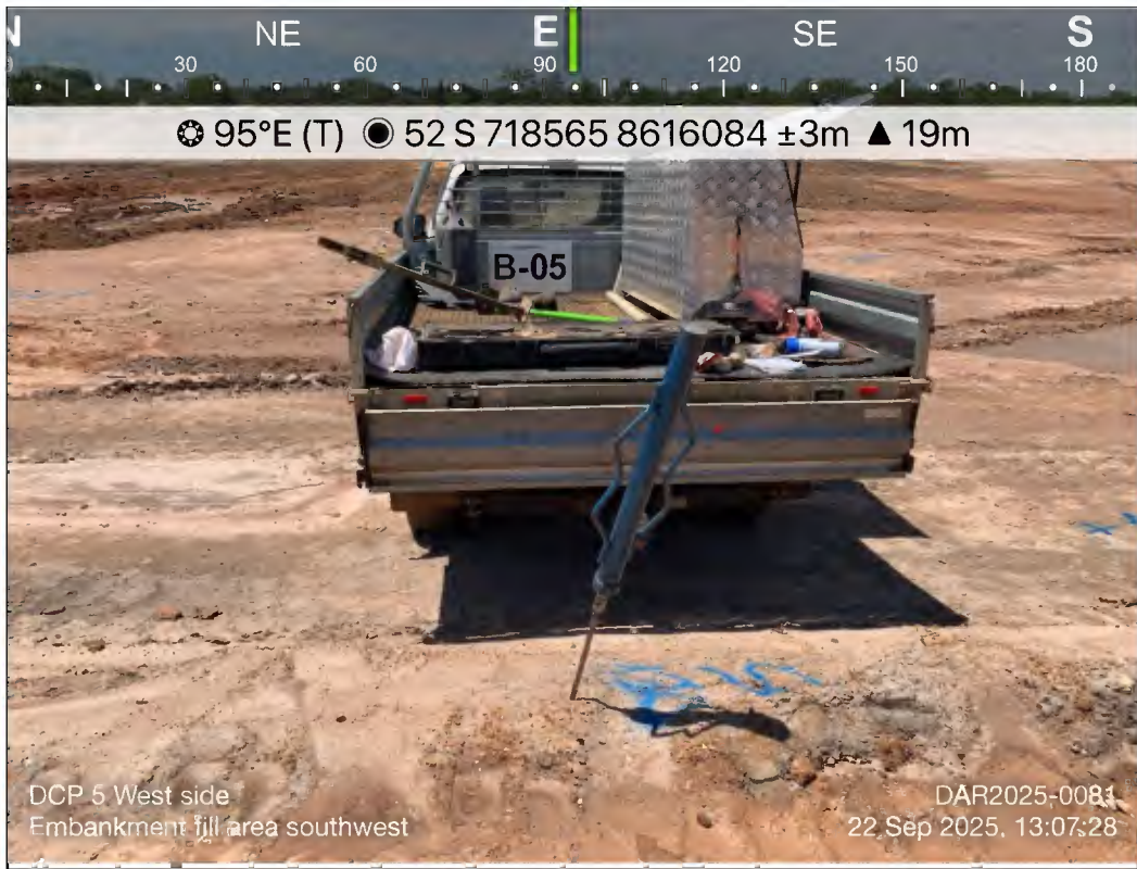
Photo 81 - DAR2025-0081_2025-09-22_DCP 5 West side_13-07-28
