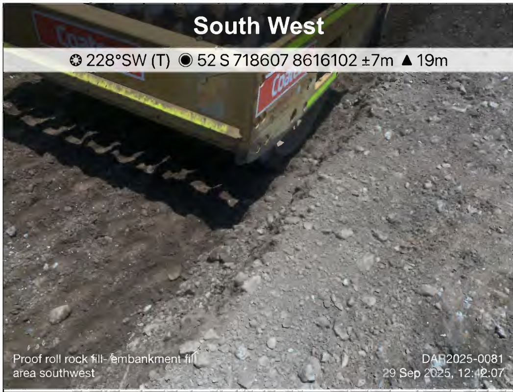
2025-0081_2025-09-29_Proof roll rock fill- embankment fill area sou
