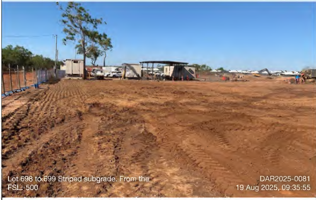
Photo 14 - DAR2025-0081_2025-08-19_Lot 698 to 699 Striped subgrade. From the FSL -500_09-35-55
