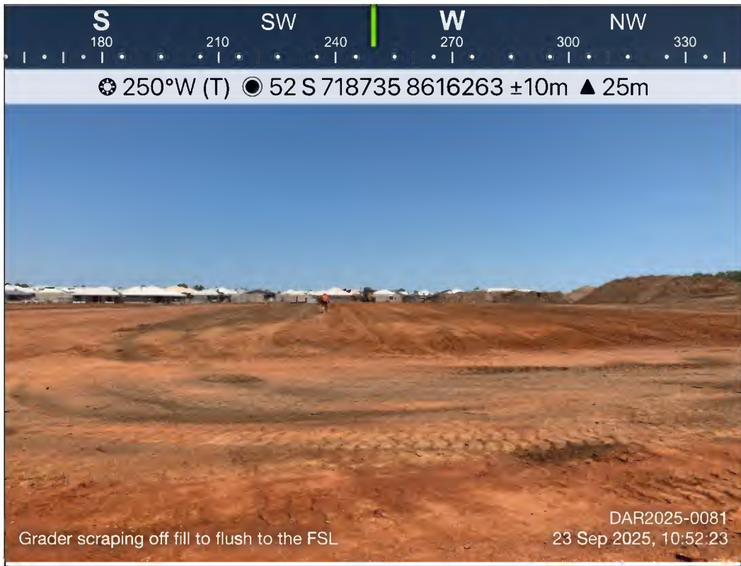
DAR2025-0081 2025-09-23 Grader scraping off fill to flush to the FSL
