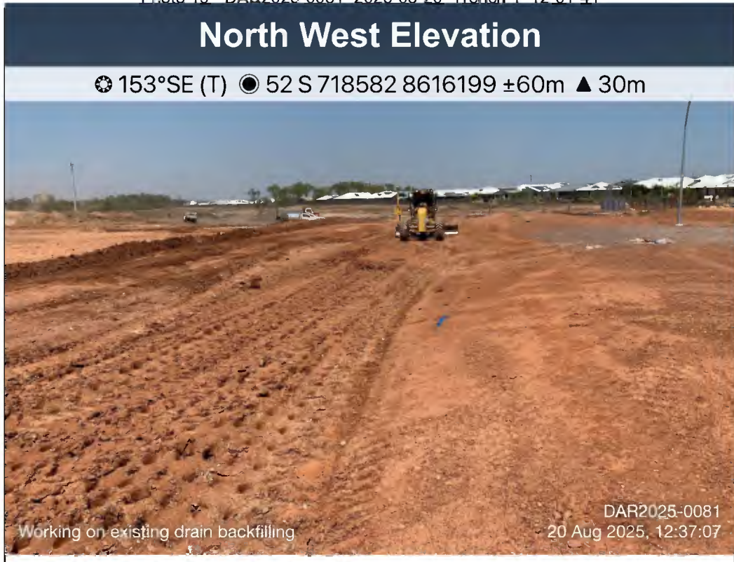
Photo 20 - DAR2025-0081_2025-08-20_Working on existing drain backfilling_12-37-07
