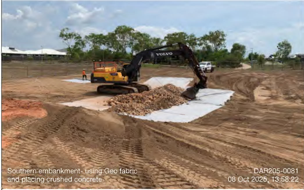
2025-10-08 Southern embankment- using Geo fabric and placing c
