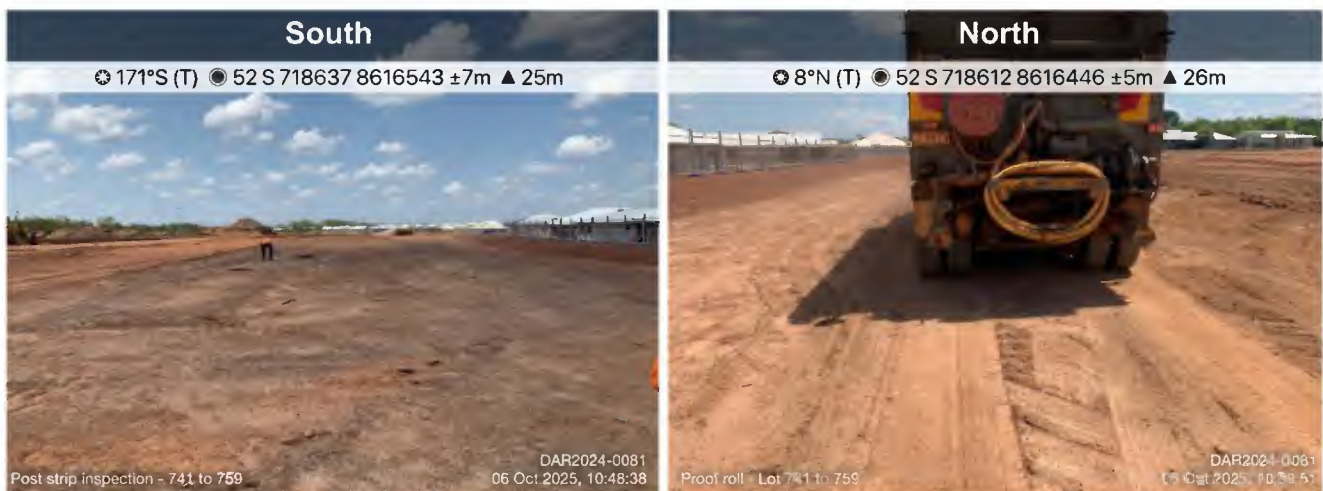
Figure 7: Post Strip area (left) followed by proof roll inspection
