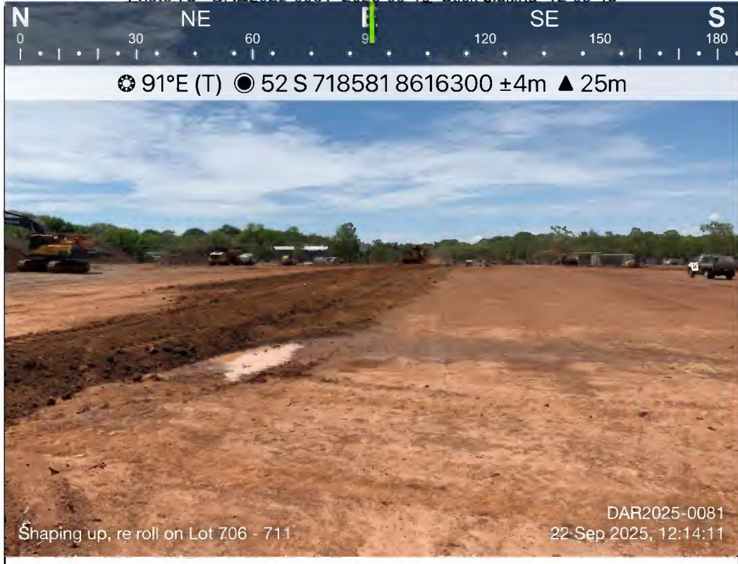
Photo 76 - DAR2025-0081_2025-09-22_Shaping up, re roll on Lot 706 - 711_12-14-11
