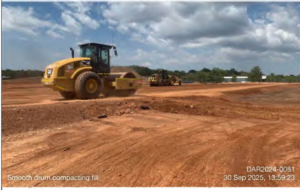
Photo 100 - DAR2024-0081_2025-09-30_Smooth drum compacting fill_13-59-23
