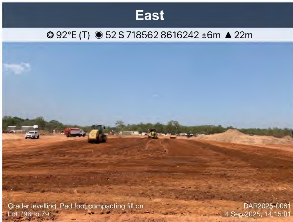
Figure 12: Level 1 site works – Typical Conditions
