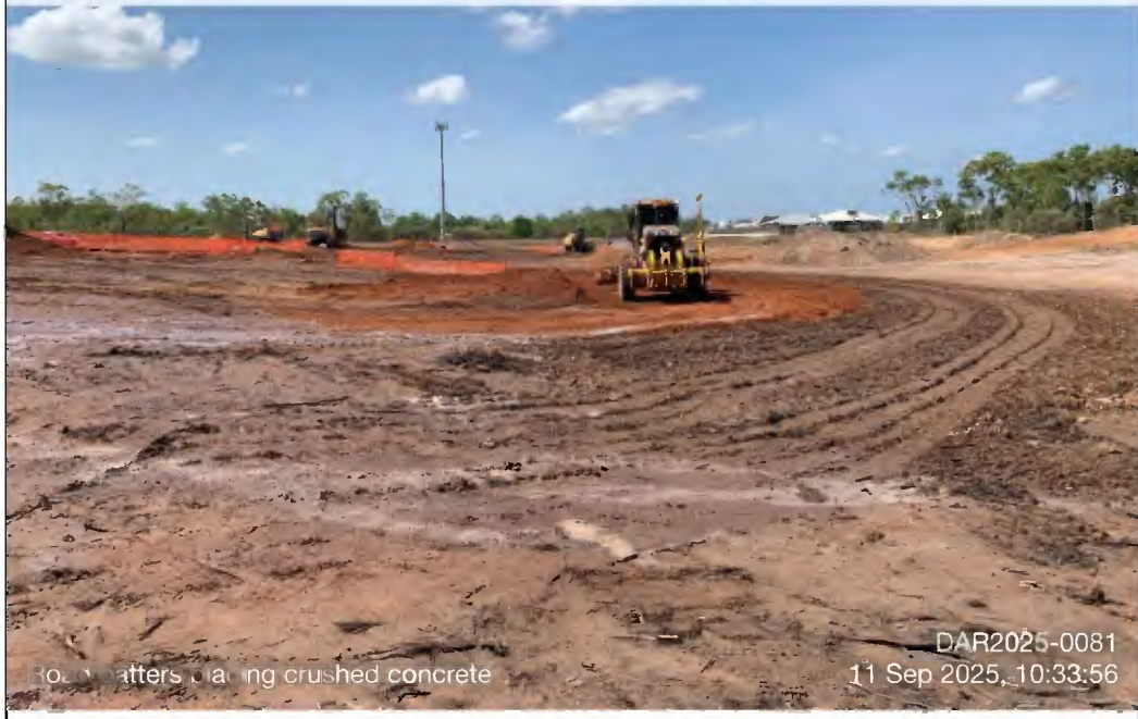
Photo 62 - DAR2025-0081_2025-09-11_Road batters placing crushed concrete_10-33-56
