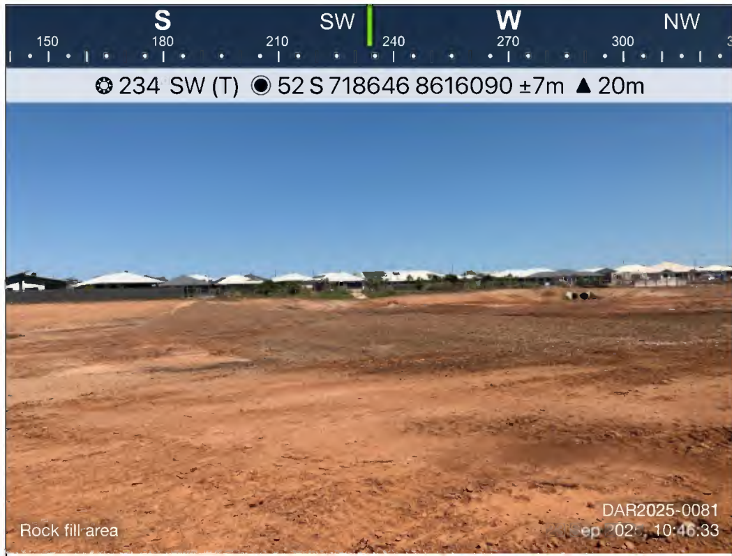
Photo 85 - DAR2025-0081_2025-09-23_Rock fill area_10-46-33
