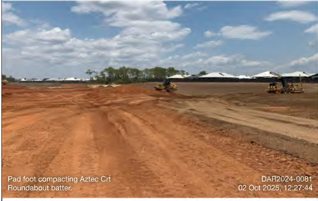
Photo 104 - DAR2024-0081_2025-10-02_Pad foot compacting Aztec Crf Roundabout batter._12-27-44
