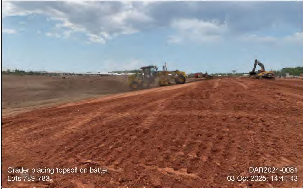
09 - DAR2024-0081_2025-10-03_Grader placing topsoil on batter_1
