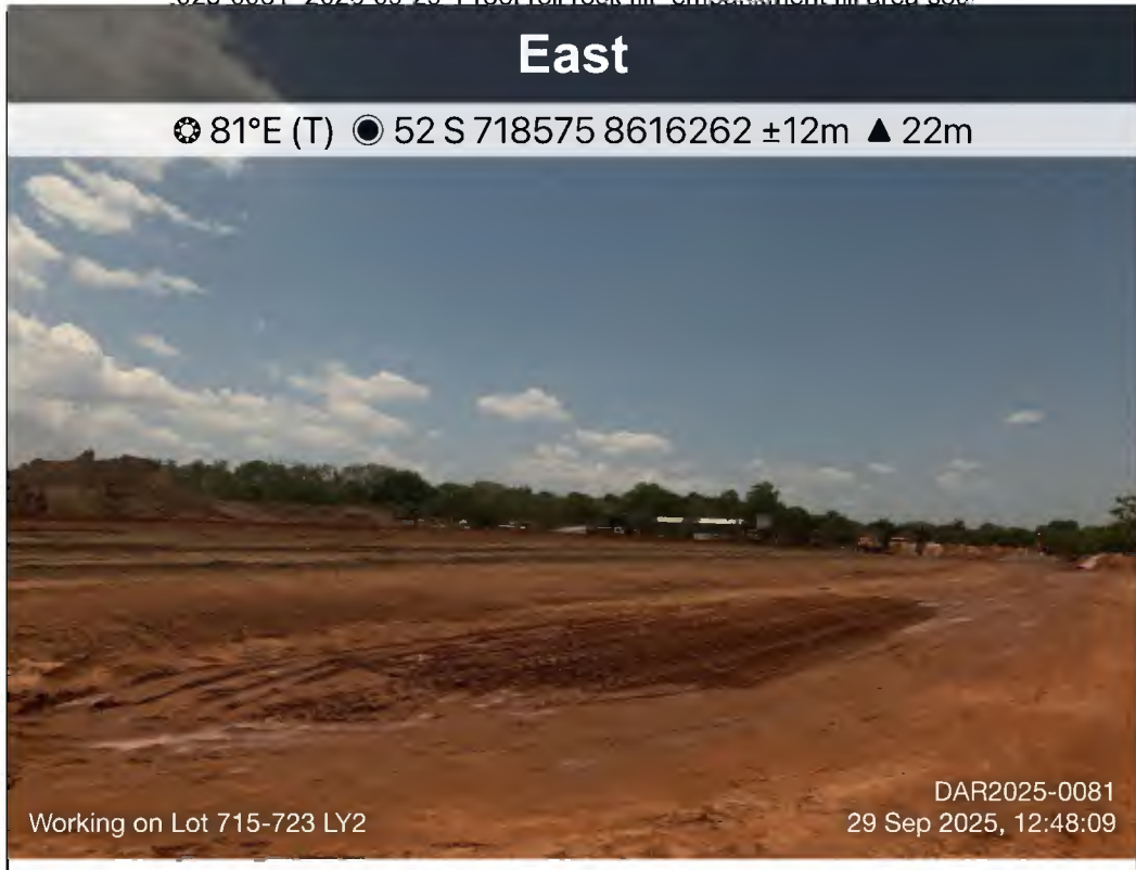
Photo 98 - DAR2025-0081_2025-09-29_Working on Lot 715-723 LY2_12-48-09
