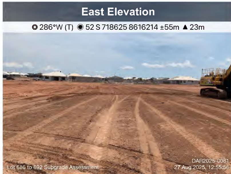
Figure 6: Site overview at Subgrade post-strip
