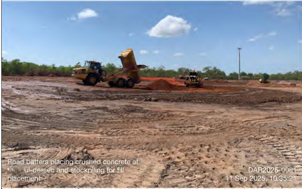
-11 Road batters placing crushed concrete at the Cul-de-sec and st
